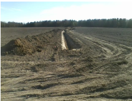
Harnett County SWCD staff provided technical assistance to a local farmer to install this V-ditch and drain tile.
