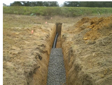
Harnett County SWCD staff provided technical assistance to a local farmer to install this V-ditch and drain tile.
