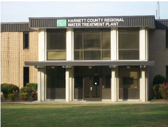
Water Plant Main Building with new signage
