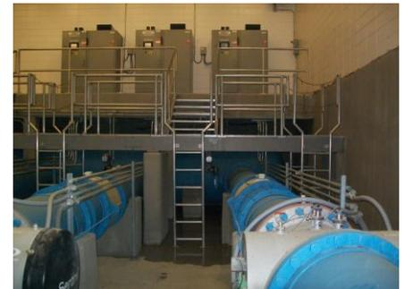
In the Calgon Carbon Corporation's Sentinel UV Disinfection System, a high-powered lamp emits UV radiation through a quartz sleeve into the water. High Energy light photons are absorbed by DNA and RNA in micro-organisms (ie. Protozoan, bacteria, viruses, Cryptosporidium parvum and Giardia) causing cross-linking of the double helix strands which prevents strands from splitting and replicating. Cells that cannot replicate are unable to infect.
