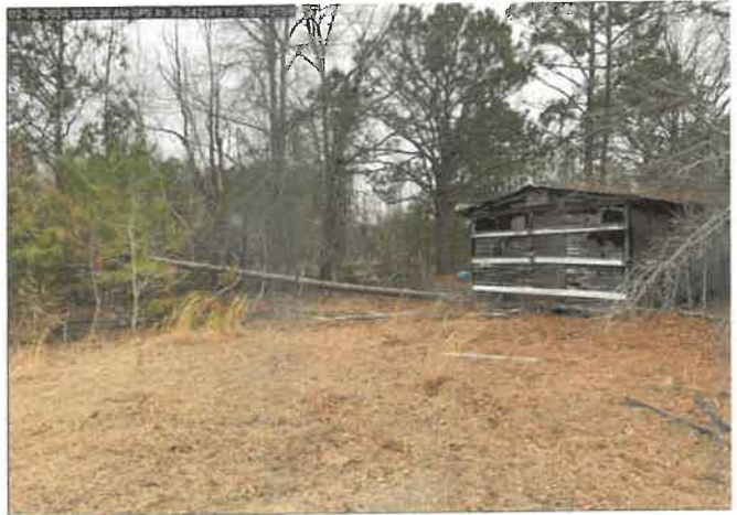
Site View Abandoned Structure
