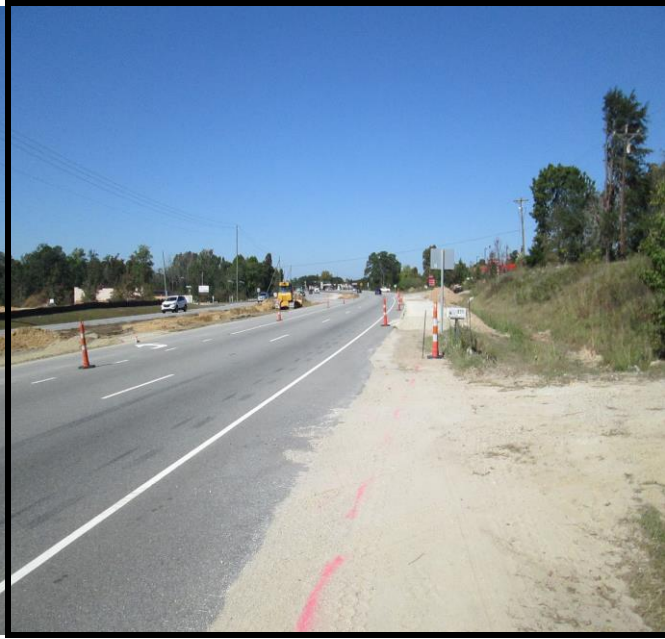
Site view along Northbound NC 24-87
