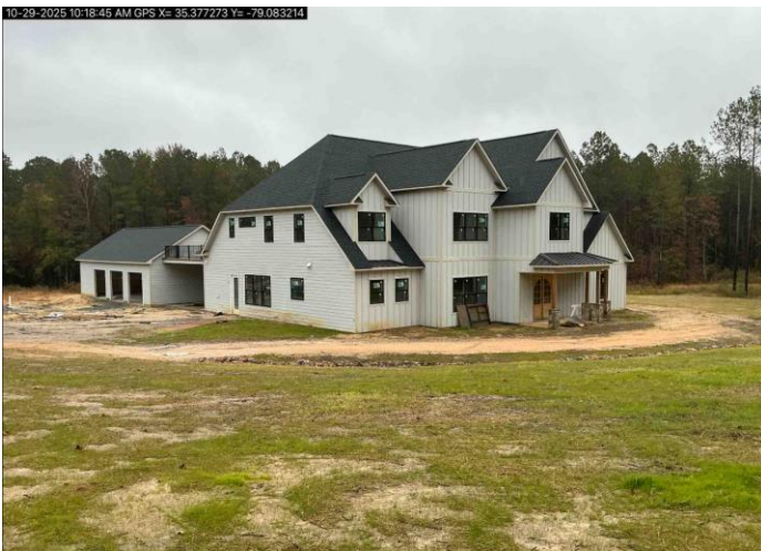
Residential Structure Under Construction
